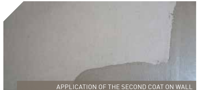
APPLICATION OF THE SECOND COAT ON WALL
